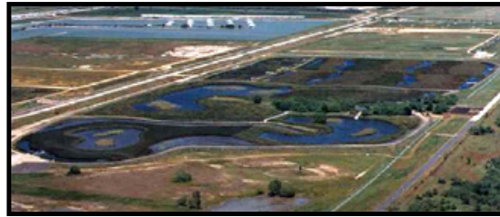
Aerial view of the wetland
