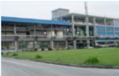
生产基地内的废水处理装置 Onsite waste water treatment plant
