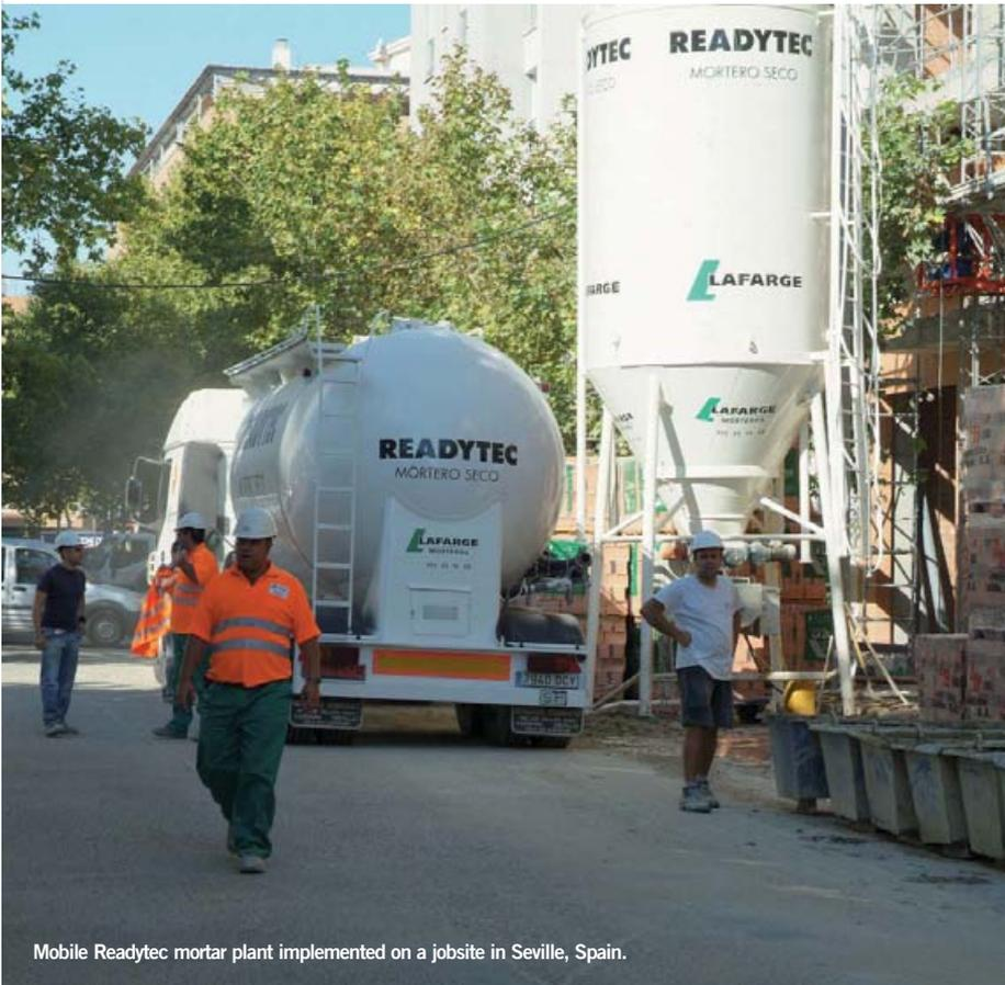
Mobile Readytec mortar plant implemented on a jobsite in Seville, Spain.
