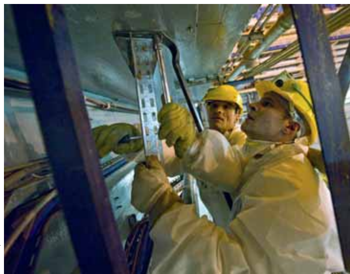
Chooz A nuclear power plant: decommissioning operation.
