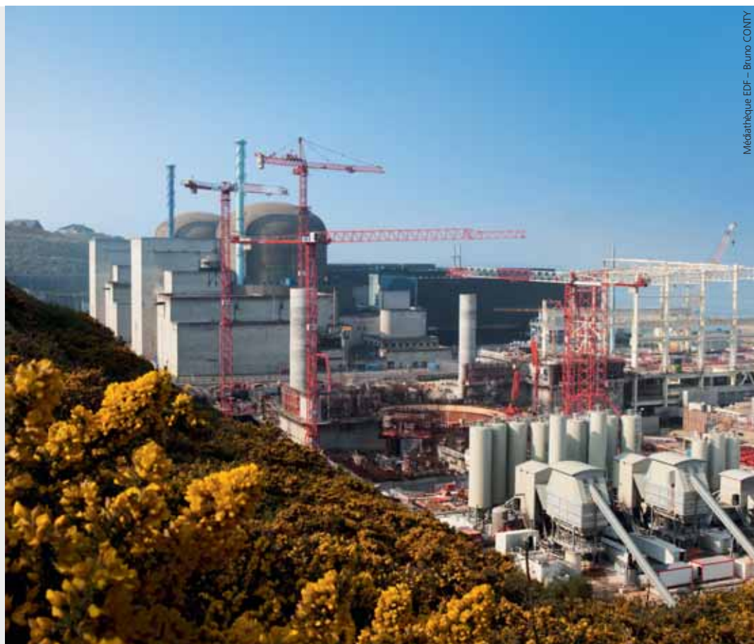
EPR construction site at Flamanville 3 (February 2009).
