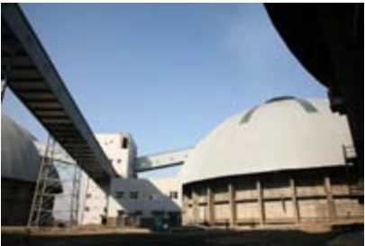
八一钢铁全封闭原料筒仓
