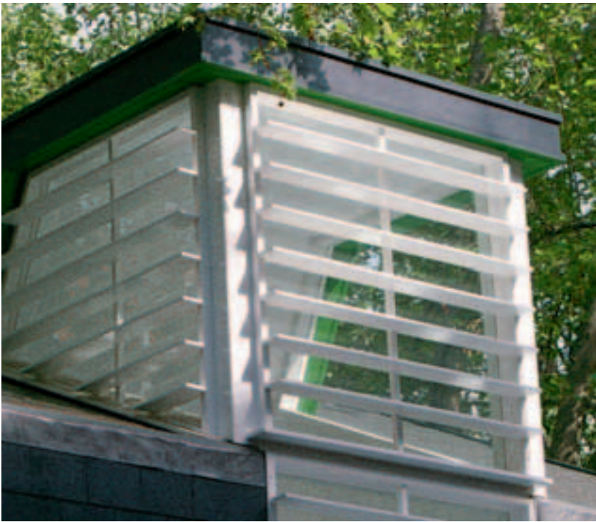
IMAGE: VENTILATION VIA CONNECTIVITY BETWEEN THE OCCUPIED OPEN PLAN SPACE, THE STAIRWELL AND THE ROOF LANTERN ENSURE OPTIMUM AIR CIRCULATION
