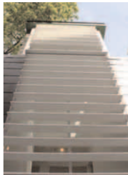
IMAGE: DESIGNING HOMES FOR A CHANGING CLIMATE - 'PUSHED IN' BAYS ON THE SOUTH AND WEST MAXIMISE SHADE. THE LANTERN PROVIDES MAXIMUM SOLAR CONTROL
