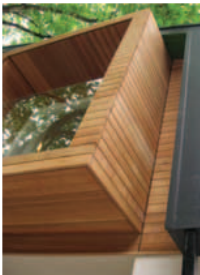
IMAGE: DESIGNING HOMES FOR A CHANGING CLIMATE - 'PUSHED IN' BAYS ON THE SOUTH AND WEST MAXIMISE SHADE. THE LANTERN PROVIDES MAXIMUM SOLAR CONTROL
